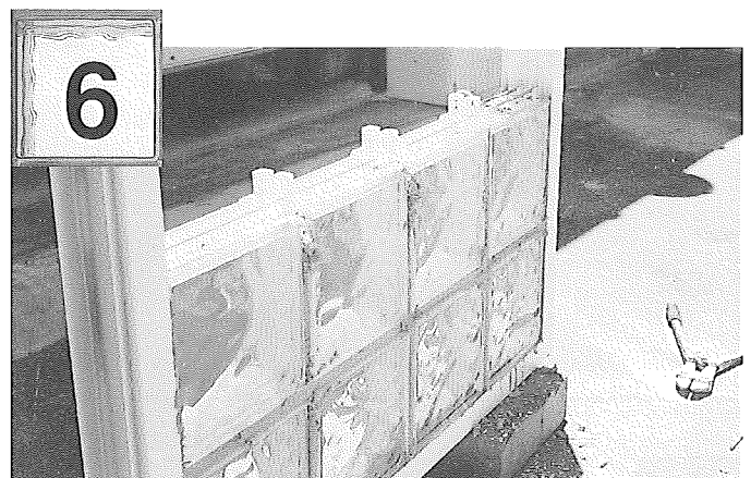
Repeat for second course using straight connectors with jamb connectors at each end.
